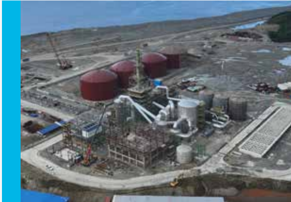
Acid Plant and Alkali Tank
