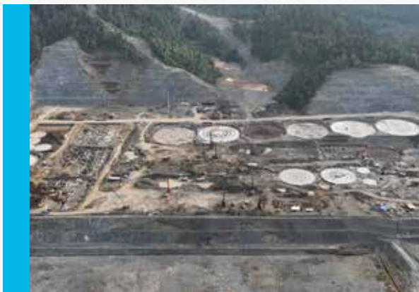
HPAL and Post-Process Area
