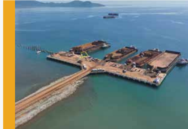
Jetty and Ore Barging Activities
