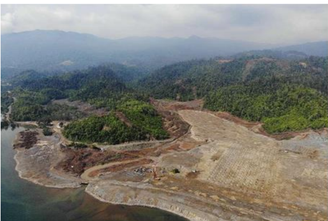
Site Clearance at Slag Yard and LNG Storage Area
