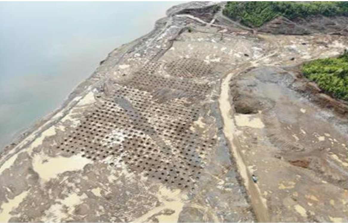
Dynamic Compaction at LNG and Power Plant
