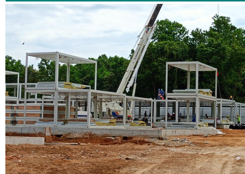
Site Office & Camp
