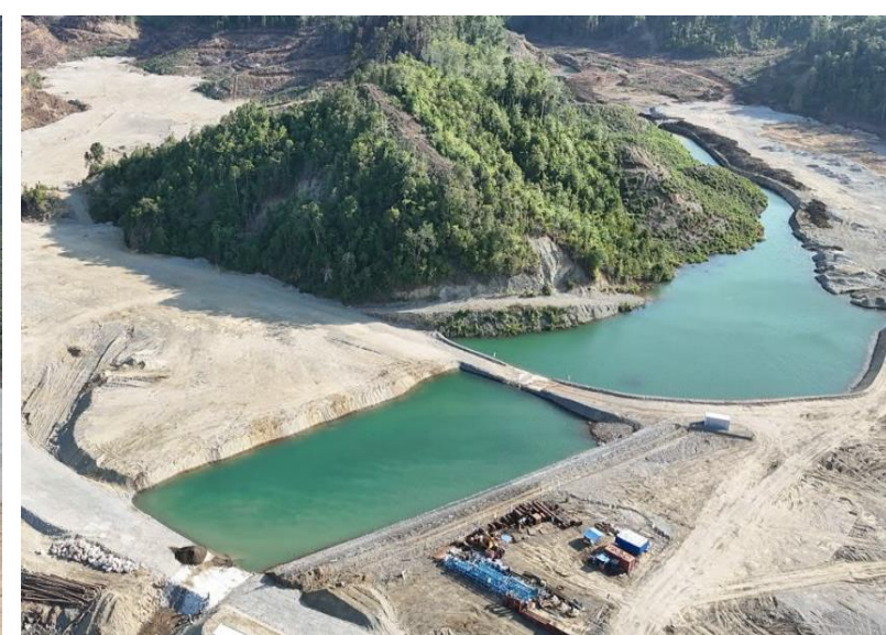
Water pond for construction
