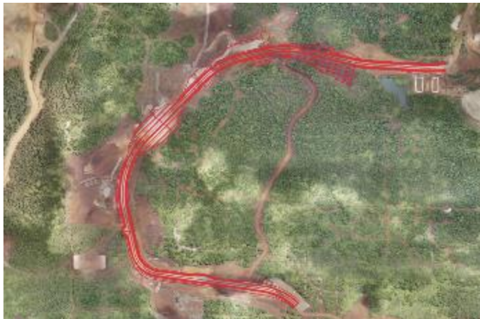
MHR STA 6+000 to 6+850 Progress 54.00%
