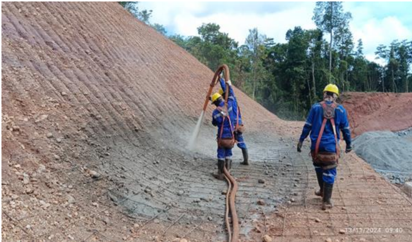
Slope Protection (Shotcrete) – KM 5 SAR
