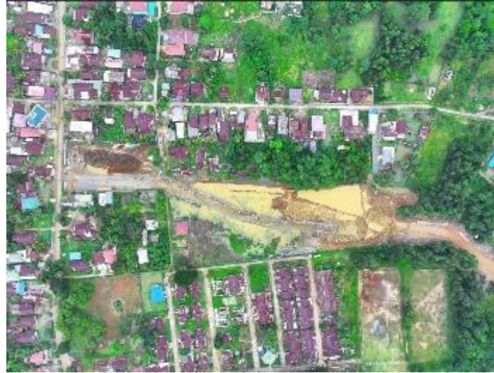
NAR PHASE-2 (STA 0 to STA 0+400) Progress 61.24%
