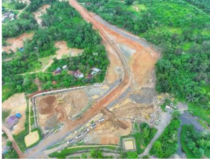
NAR PHASE-1 (STA 0+850 to STA 1+450) Progress 95.94%
