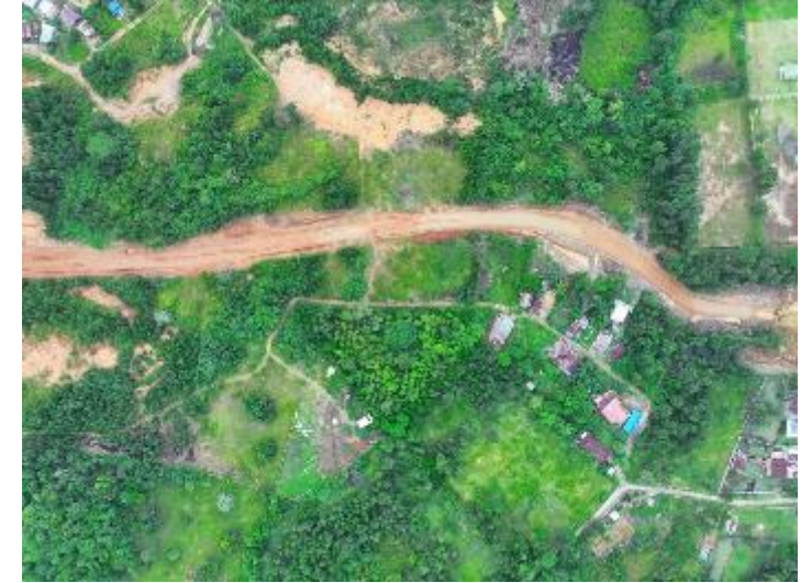
NAR PHASE-3 (STA 0+400 to STA 0+850) Progress 88.01%
