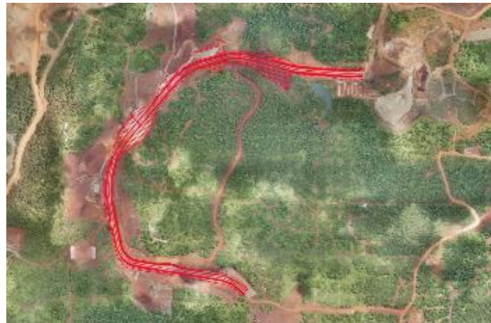
MHR STA 6+850 to 8+000 Progress 87.00%
