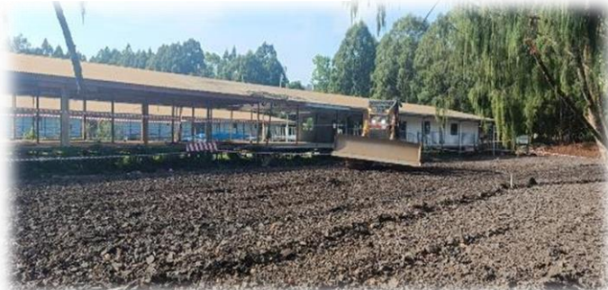
Laydown preparation for Construction Camp
