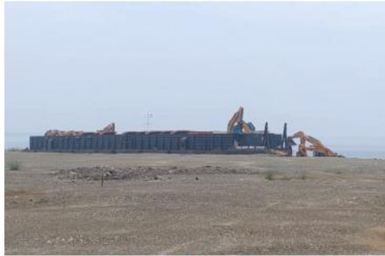
Temporary Port is Being Utilized During Mobilization
