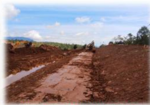
Hasan Koro-3 Stockpile Sloping Area
