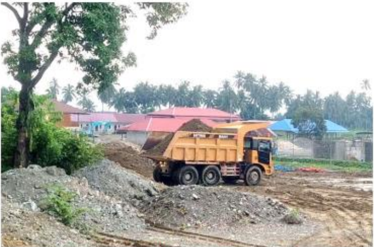
Backfill and Grading on Camp Upgrade Area
